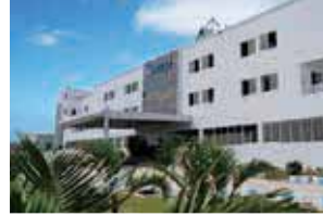
Rudrapur Plant (Green Building)
