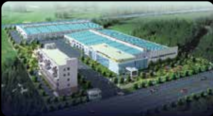
• TECHTOP Shanghai Himak Electrical Machinery Co., Ltd.
