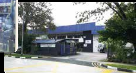
• Singapore Elektrim Techtop Motors Pte Ltd.
