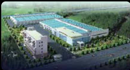
• TECHTOP Shanghai Himak Electrical Machinery Co., Ltd.
